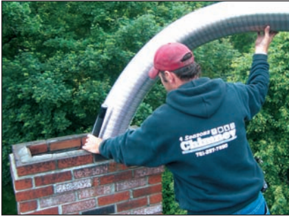
Flex liners are the most common type, and must be used for relining chimneys with offsets.
