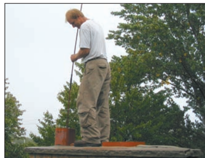
The chimney should be cleaned thoroughly before relining.
