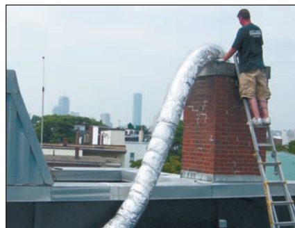
Blanket insulation must be carefully installed.
